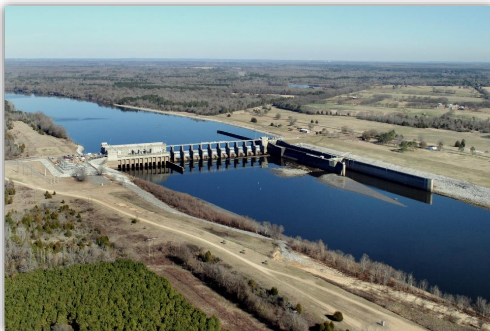
Figure 2-4 Robert F. Henry Lock and Dam
