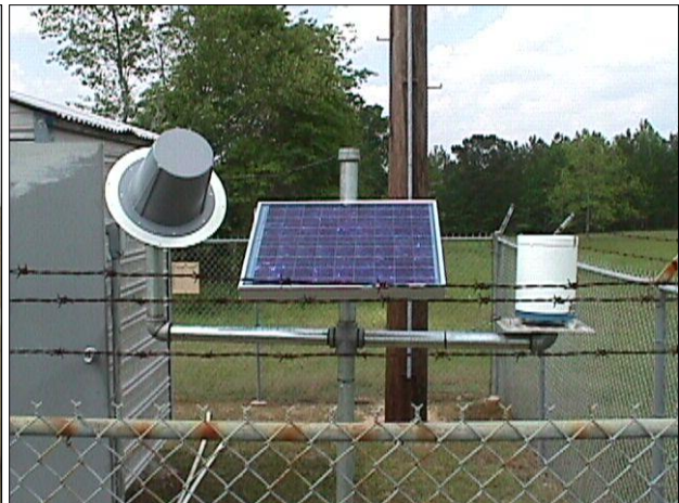
Figure 5-2 Typical Field Installation of Precipitation Gage
