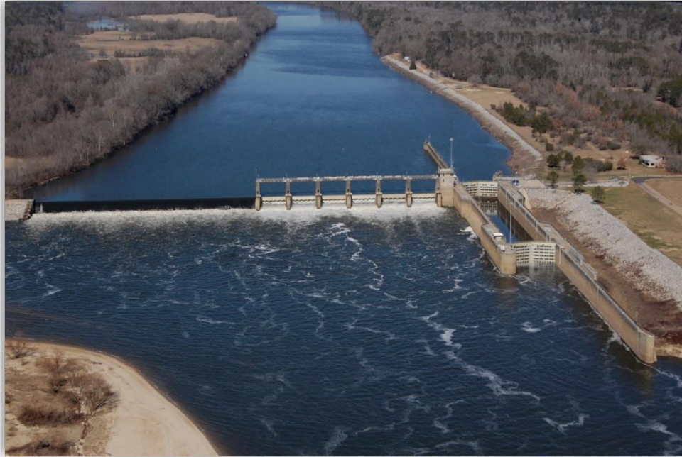
Figure 2-6 Claiborne Lock and Dam
