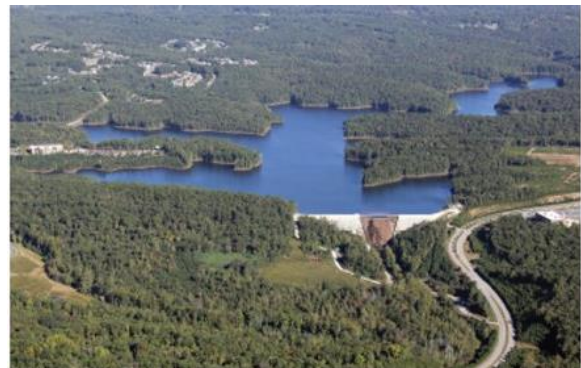
Figure 2-19 Hickory Log Creek Dam
