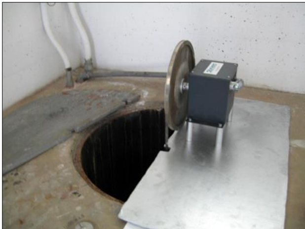
Figure 5-1 Typical Encoder with Wheel Tape for Measuring the River Stage or Lake Elevation in Stilling Well
