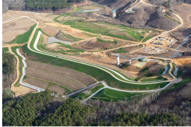
Figure 2-20 Richland Creek Dam
