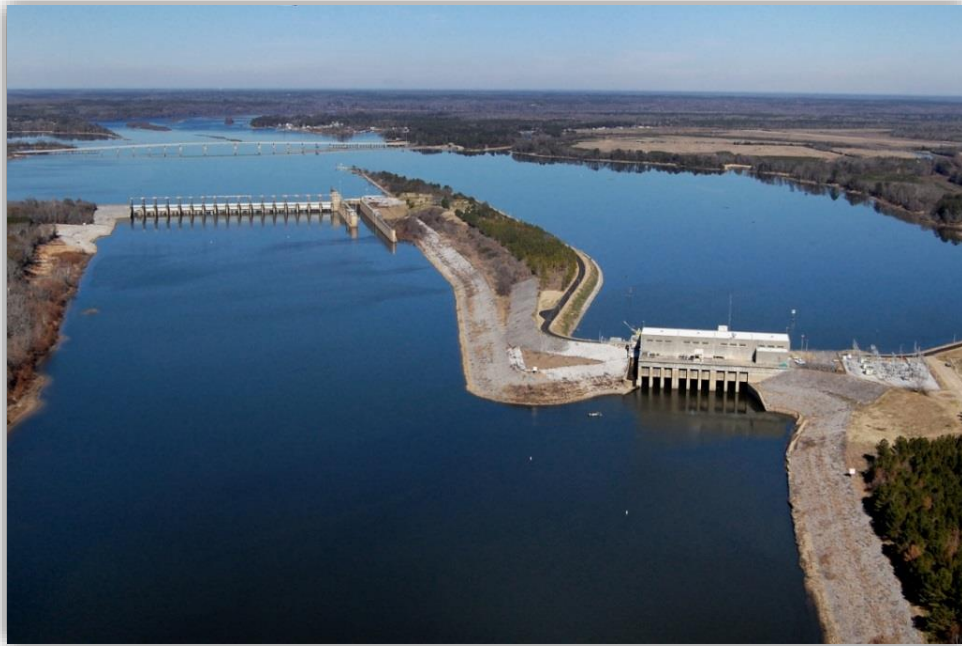
Figure 2-5 Millers Ferry Lock and Dam
