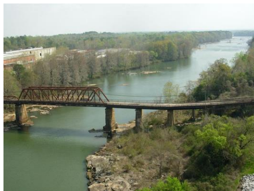
Figure 4-13 Tallapoosa River at Tallassee, Alabama
